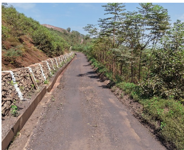
Construction of Retaining Wall & Garland Drain at the toe of waste dump during the RY
