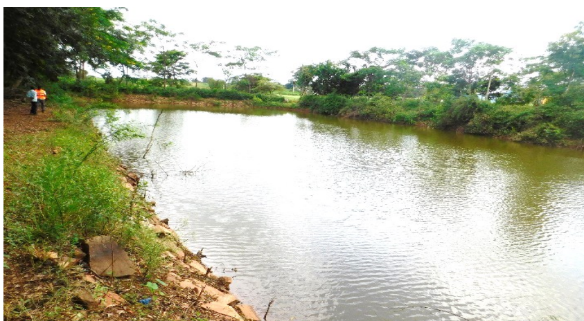
Rain water collection and harvesting pond
