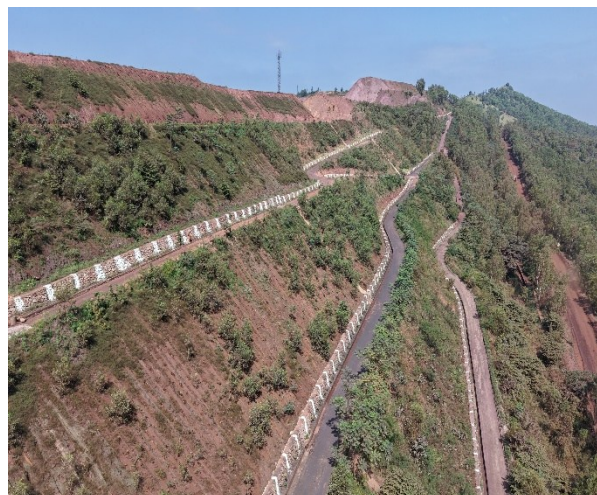
Construction of Retaining Wall & Garland Drain at the toe of waste dump during the RY
