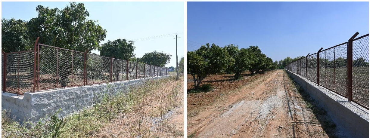
Construction of fencing at Uma Maheshwara Temple, Hireyemmiganuru
