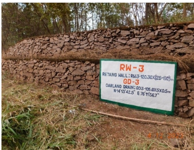
Retaining wall and garland drain as part of Soil & Moisture Conservation
