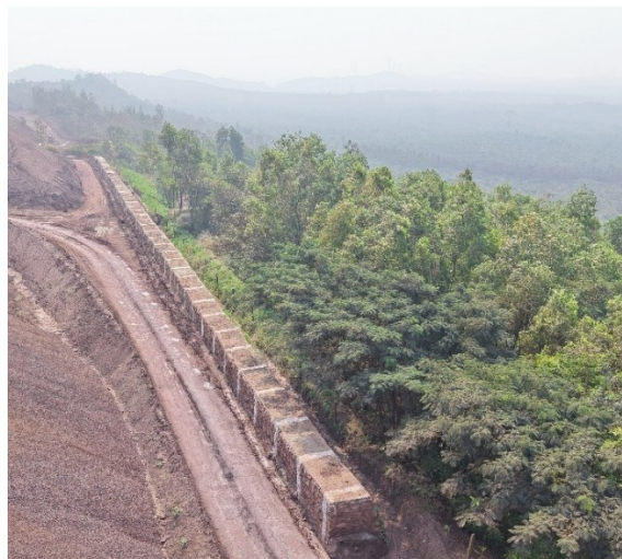
Retaining wall and garland drain as part of Soil & Moisture Conservation
