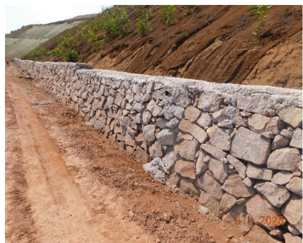
Retaining Wall at the toe of waste dump
