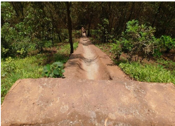
Vertical Drain, Retaining Wall & Garland Drain (work in progress) at toe of waste dump
