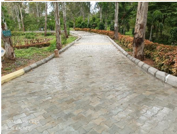
Construction of Visitor's pathway with Interlocking Pavers
