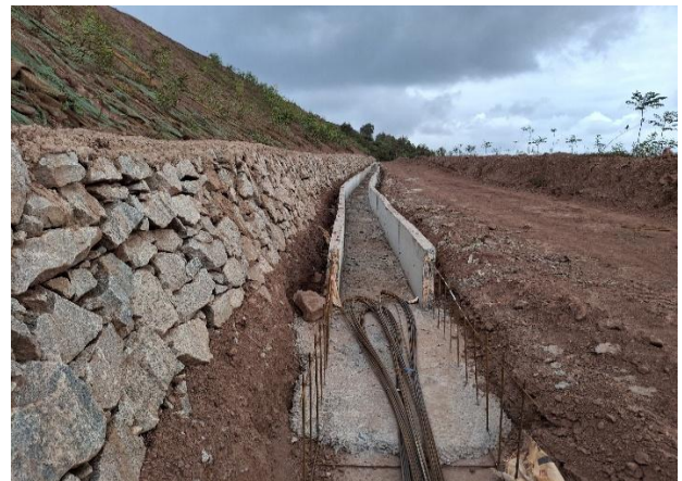
Vertical Drain, Retaining Wall & Garland Drain (work in progress) at toe of waste dump
