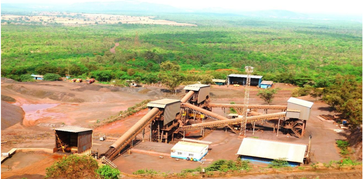
Hood cover on the conveyors of processing plant within the green ambient
