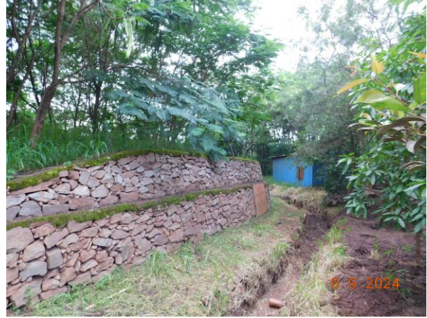
Retaining wall and garland drain as part of Soil & Moisture Conservation
