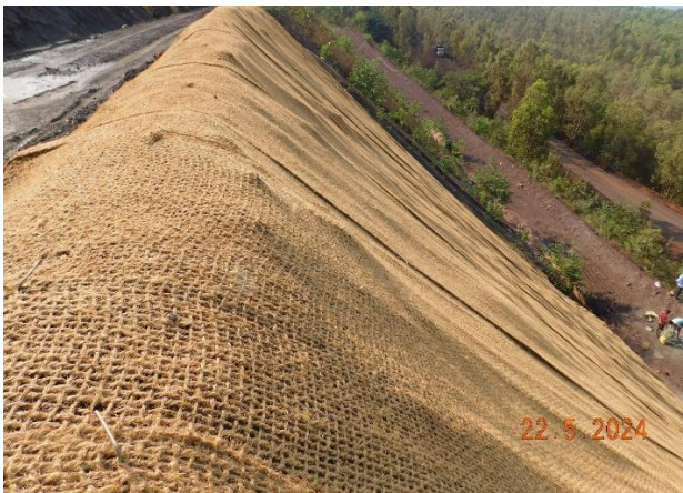
Geo textile/coir mats laid on waste dump & Dump covered by Grass
