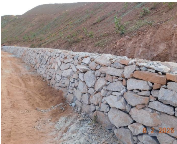
Retaining Wall at the toe of waste dump
