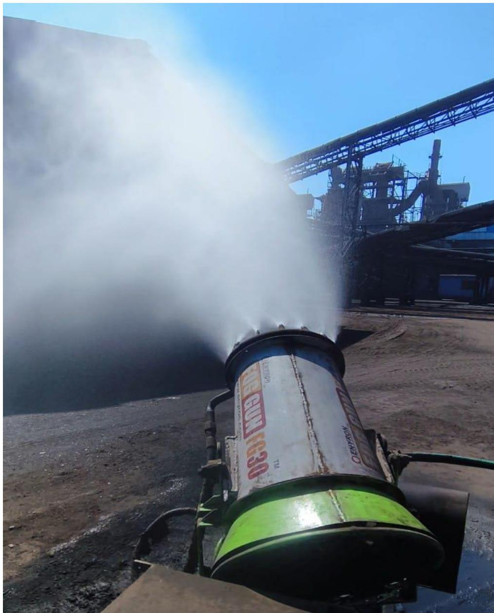
**Photos of the Dry Fog system installed at the coal and iron ore discharge points.**
