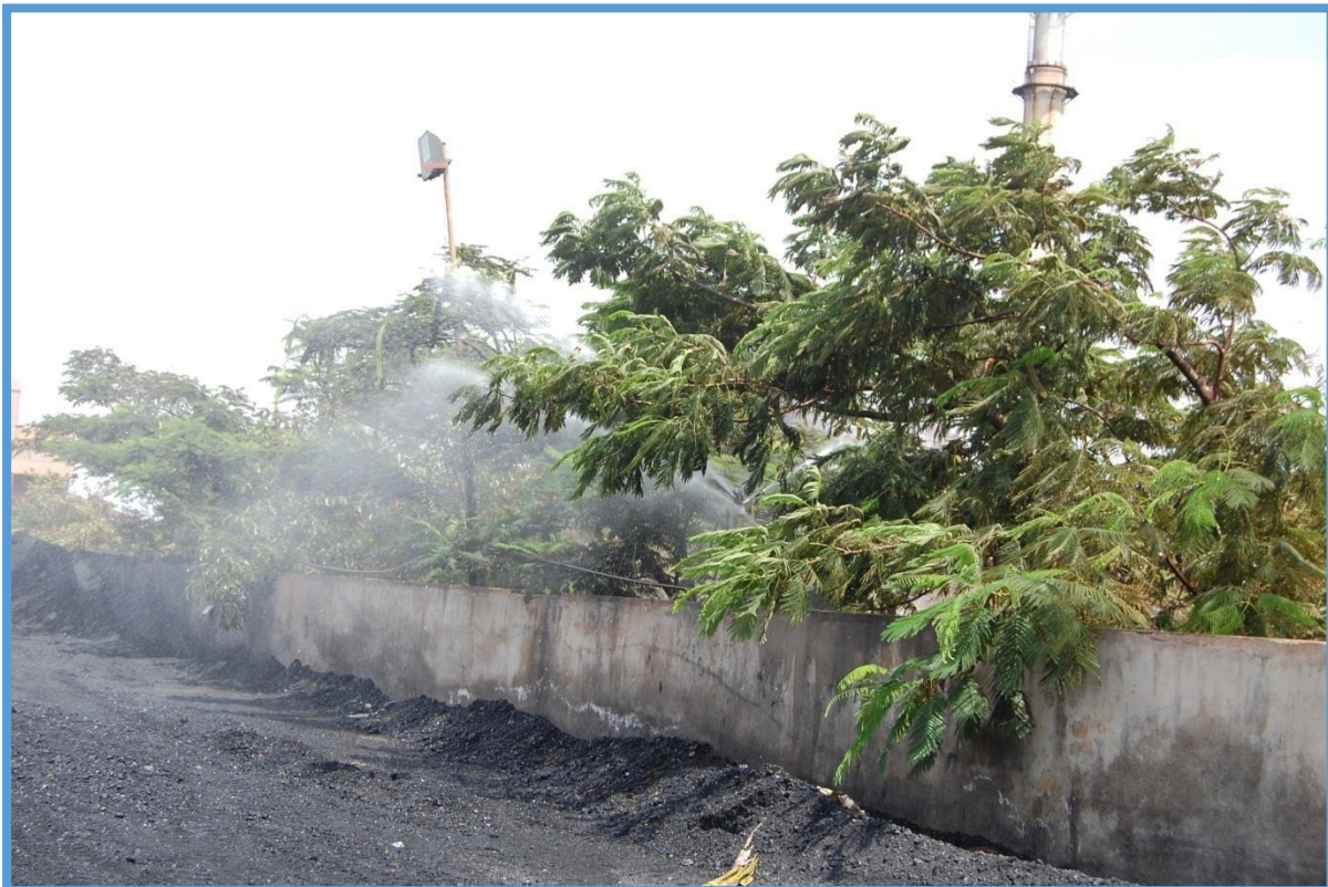
Sprinklers Installed at Bottom Ash Handling Area
