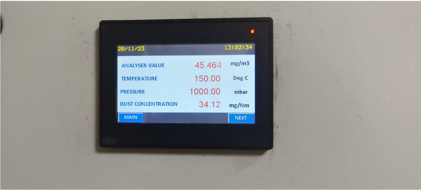
OCEMS display unit installed in our plant
