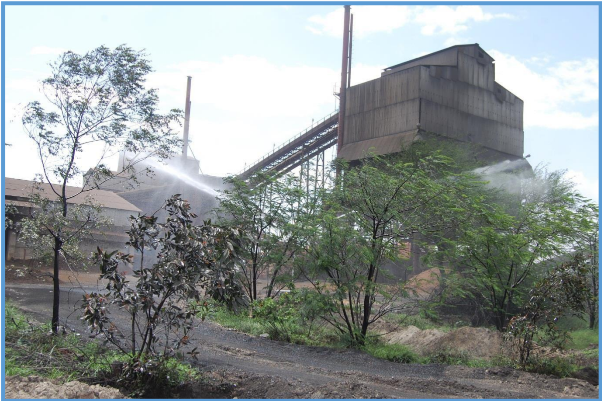
Sprinklers Installed at Bottom Ash Handling Area
