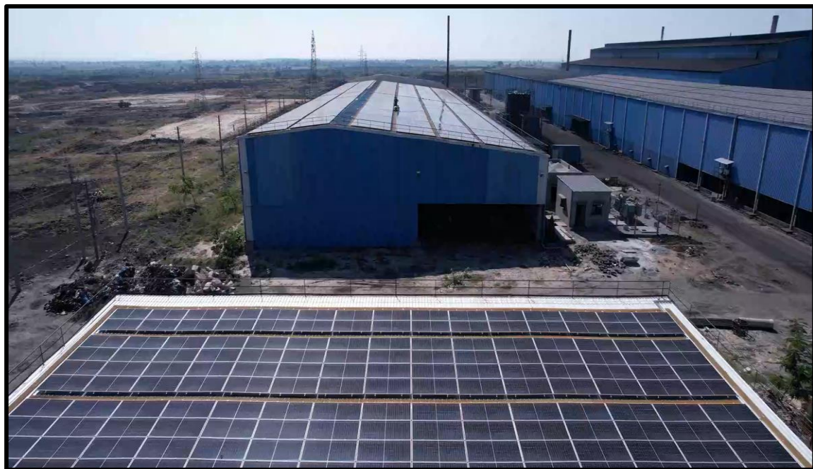
3.6MW roof top mounted solar power plant established to generate own electricity
