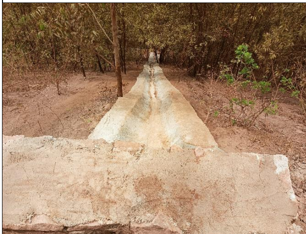
Vertical Drain on Waste Dump
