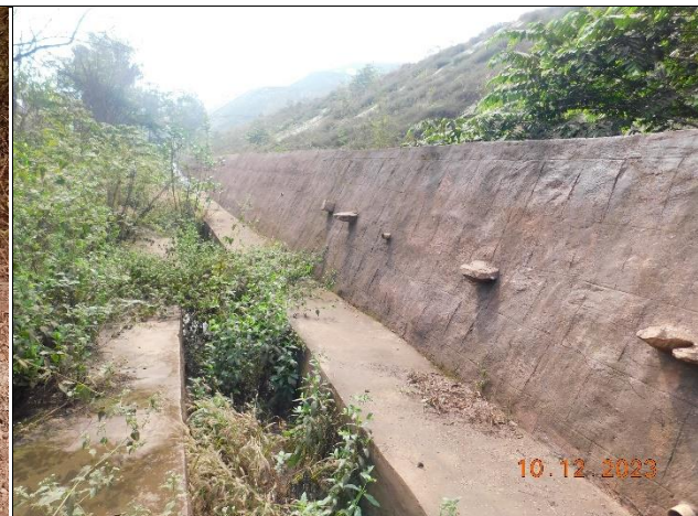
Retaining Wall & Garland Drain at toe of waste dump under progress
