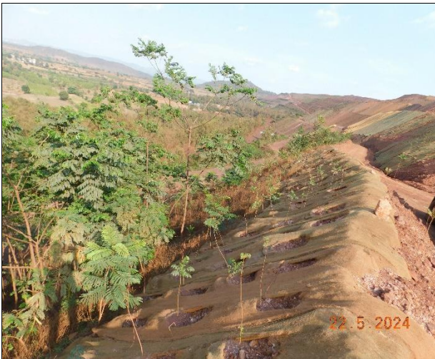
Geo textile coir mats laid on waste dump & Dump covered by Grass
