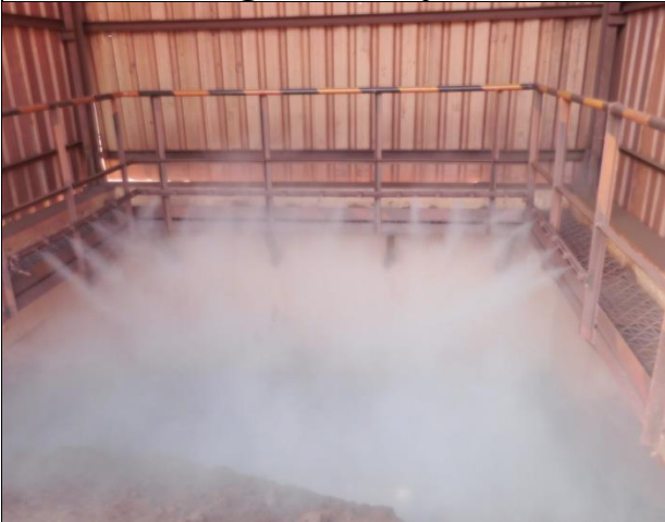
Dry fog dust Suppression system at the Input of Mineral Processing Plant
