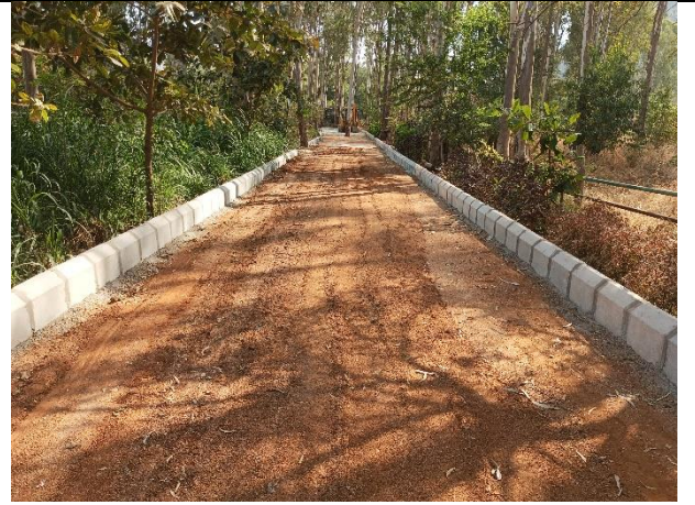
Construction of Visitor pathway with Interlocking Pavers and Kerb stones at Adumalleshwara Mini Zoo, Jogimatti, Chitradurga.
