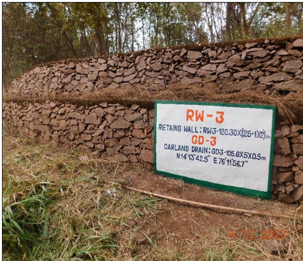
Retaining wall and garland drain, enrichment plantation as part of reclamation
