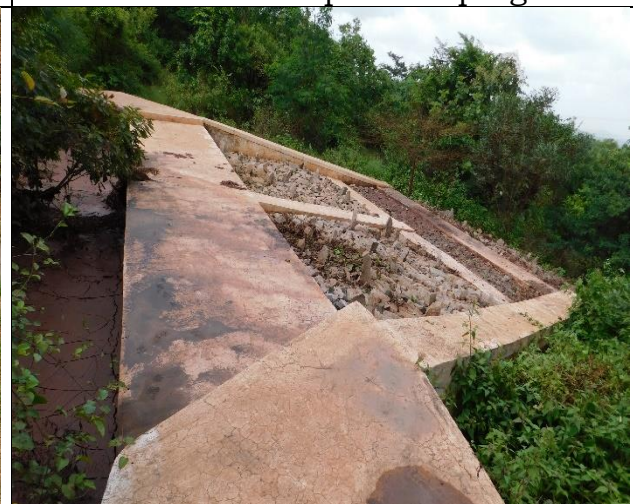
Reconstruction of Check Dam outside the lease area
