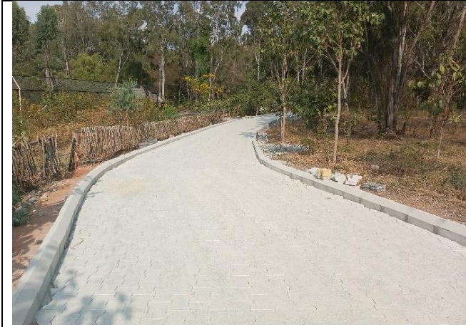
Construction of Visitor pathway with Interlocking Pavers and Kerb stones at Adumalleshwara Mini Zoo, Jogimatti, Chitradurga.
