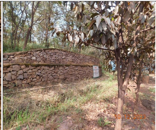
Retaining wall and garland drain, enrichment plantation as part of reclamation
